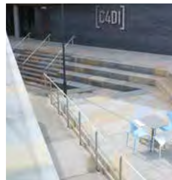
Centre for Digital Innovation, Hull (Bespoke cut sandstone paving, copings and steps)
