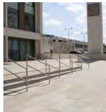
District Police Headquarters, Leeds (Bespoke cut paving, tactile paving and steps with granite inserts)
